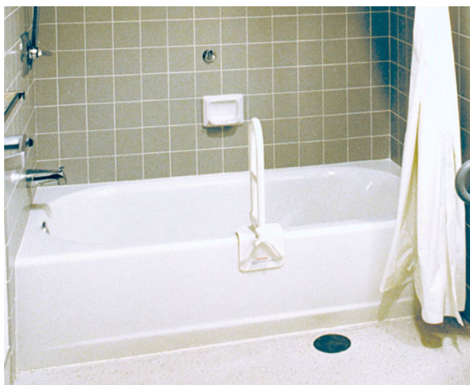
▲ Safety features such as handrail on bathtubs assist in preventing client falls.
