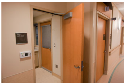
▲ Entrance to Negative Pressure isolation room and the adjoining Anteroom.
